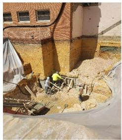
Then they began digging for the installation of the elevator. This will be a 16' hole so the elevator may reach the gym level and the pit below the elevator for service.
