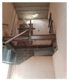
Monarc began with the demolition of restrooms, and the removal of the external and internal stairways.
