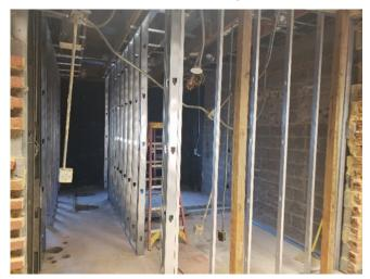
Framing out of the new bathrooms and preparations for plumbing has begun.
